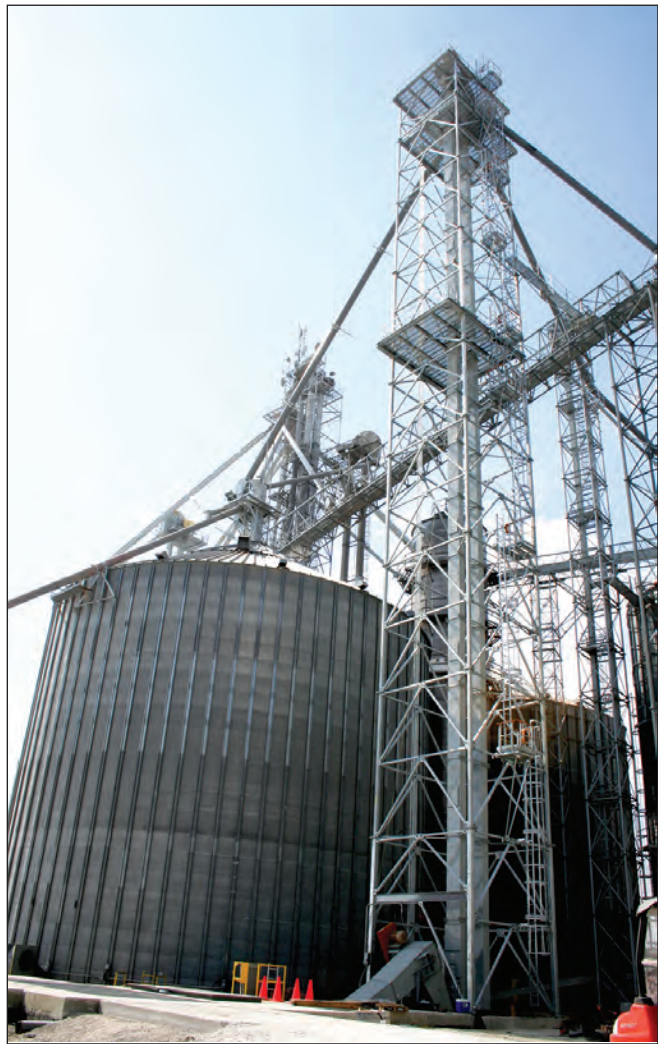
FS Grain in Mazon added a leg to a storage tank capable of moving 20,000 bushels an hour. The new leg and loading pit is the third pit now available to area farmers at the elevator, just in time for this year's harvest. The Paper photo
