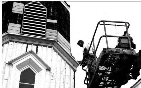
VISSERING CONSTRUCTION workers continue to replace rotten wooden sections of the Pioneer Gothic Church steeple. Work is expected to be completed in early October.
