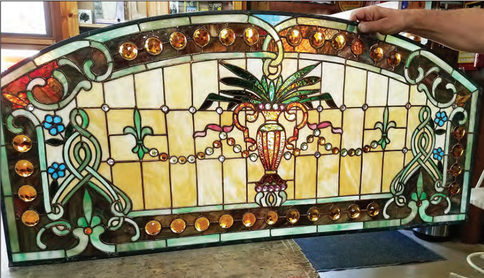
THIS REPAIR JOB FOR a stained glass window containing 498 glass pieces included 40 broken pieces to be replaced. The 1920s style window is from a house in California, restored by Tom Perkins of Gardner. The Paper photo
