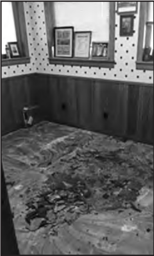
125 YEARS WORTH of glue was caked onto the original maple flooring at the Dwight historic depot, now the home to the Dwight Historical Society. This shows the floors before they were restored. submitted photo above
