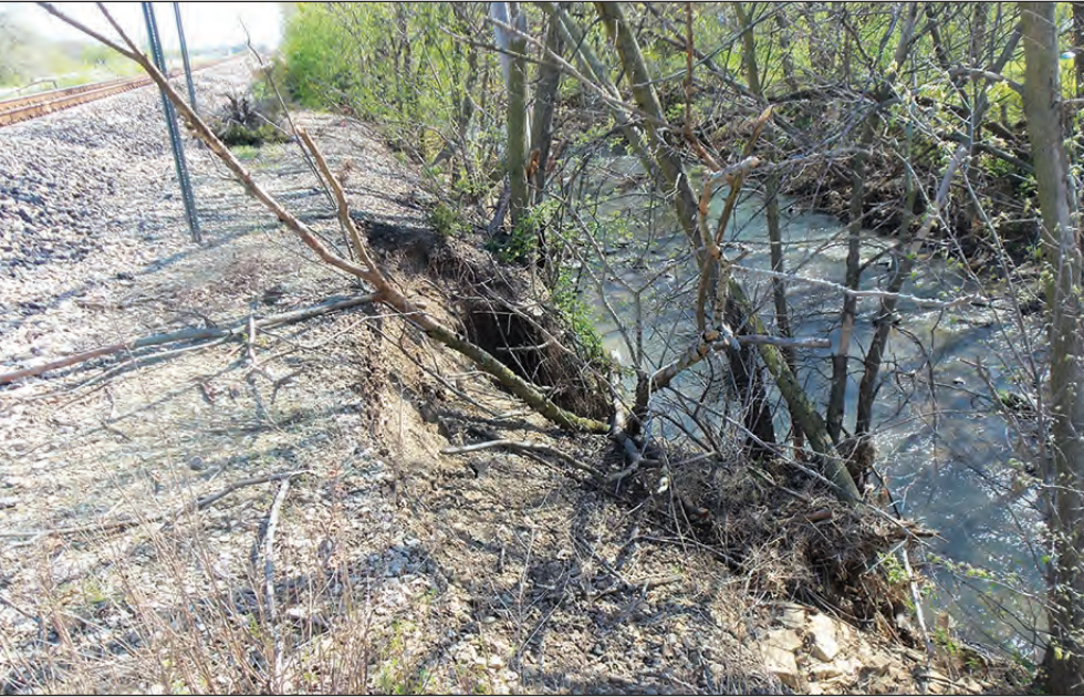
IN MAY OF 2013, the banks of the Gooseberry Creek west of Seminole had eroded, causing Ron Simmons alarm as the banks were close to a railroad track.
