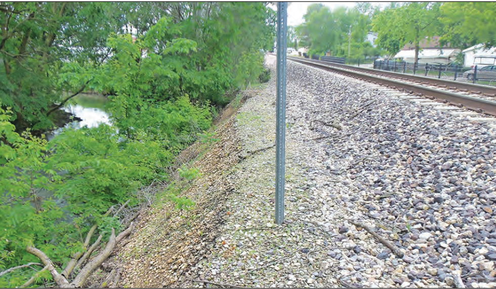
THIS PHOTO TAKEN IN May of this year clearly shows how the banks of Gooseberry Creek have eroded over the years, creeping dangerously closer to the Union Pacific Railroad tracks.
