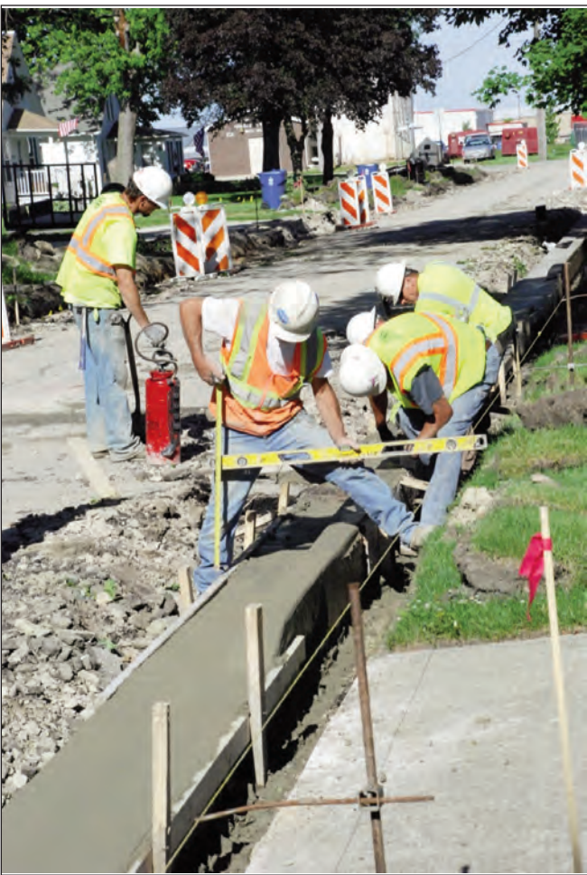
THE MARVELOUS CONCRETE CURB FORMING MACHINE still requires some manual labor to smooth out a few irregularities. Above, workers from D Construction add finishing touches to the curb being poured along West Delaware Street in Dwight last week. Twenty-nine blocks have been designated for new pavement in Dwight's Phase I of residential street repaving. The Paper photo
