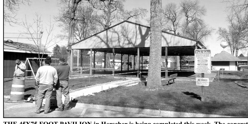
THE 45X75 FOOT PAVILION in Herscher is being completed this week. The concrete floor and ramp have been poured. The pavilion is between the "big stand" and the baseball diamond.
