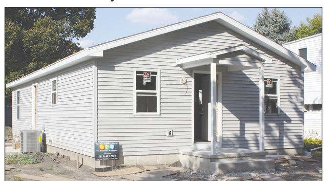
Habitat for Humanity home in Dwight.
