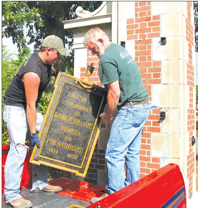
THE GATES AT RENFREW PARK, Dwight, were recently refurbished as an IMPACT Dwight project. Tech-Ni-Kolor Autocrafters soda-blasted and power-washed the gates, cleaned, clear-coated and touched up the gate plaques. The plaques, which honor David McWilliams as the park's benefactor, had become green with oxidation and age and had probably not been cleaned since they were originally installed about 100 years ago. They were re-installed September 15 by Tech-Ni-Kolor's Nathan Bissee, left, and Larry Seabert. More photos on page 2.
