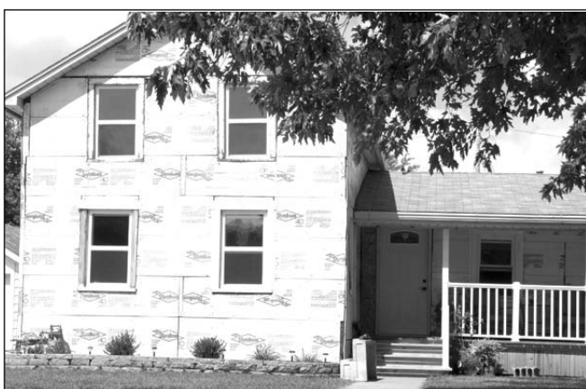
A HOUSE ON SEMINOLE STREET IN DWIGHT receives a face-lift.
