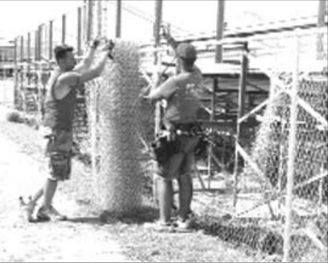
NEW FENCING was being rolled out August 19 around Oughton Athletic Field at DTHS by workers from Ifft Quality Fencing. The fence around the field was damaged by the tornado that swept through on June 5.
