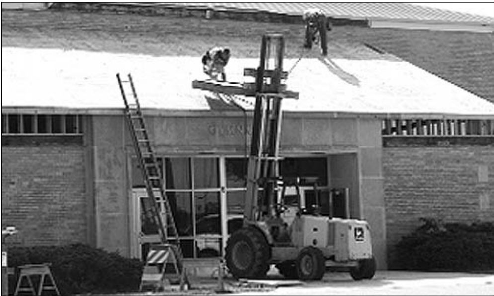
WORKERS REPAIR THE ROOF above the Dwight Township High School Kresl Gymnasium entrance August 19. The roof was damaged during the June 5 tornado.
