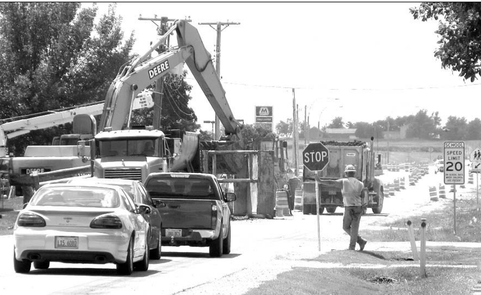
TRAFFIC IN SAUNEMIN waits for the go-ahead from a construction worker July 7. Road construction is underway on Route 116 through the village.
