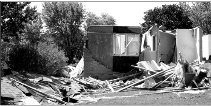
Aerial photo of Janet Kresl's house at 312 Linden and below left, the front view of the Kresl house and below right, a section of the roof lays in her backyard. The garage of the Kresl house was exposed when the tornado tore down an exterior brick wall and ripped the roof off the house.
