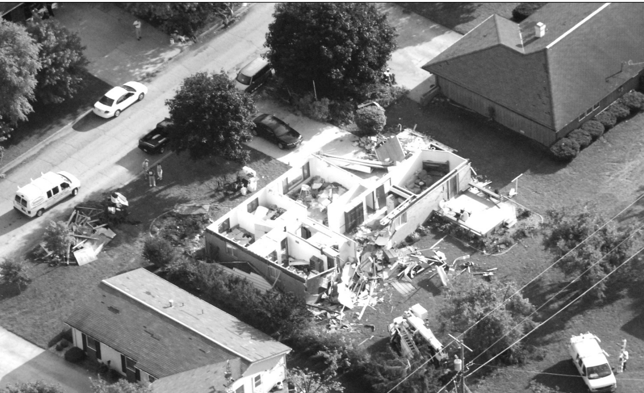
Aerial photo of Janet Kresl's house at 312 Linden and below left, the front view of the Kresl house and below right, a section of the roof lays in her backyard. The garage of the Kresl house was exposed when the tornado tore down an exterior brick wall and ripped the roof off the house.
