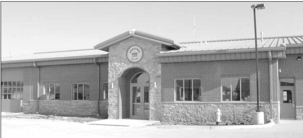
CONSTRUCTION IS NEARING COMPLETION of the Herscher Fire Department headquarters on East Myrtle Street. The move is scheduled to be made soon from the old station on Main Street. Village officials are still pondering changing the zoning so the fire department can sell the old building.
