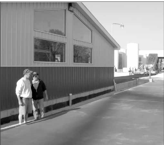
WORK HAS BEEN GOING ON for the past seven weeks to renovate the facilities at Herscher Grain. Shown here are the new scale house and new scales, which will be able to handle twice the weight of the old scales. In the background, workers put down asphalt for the facility's open lot.
