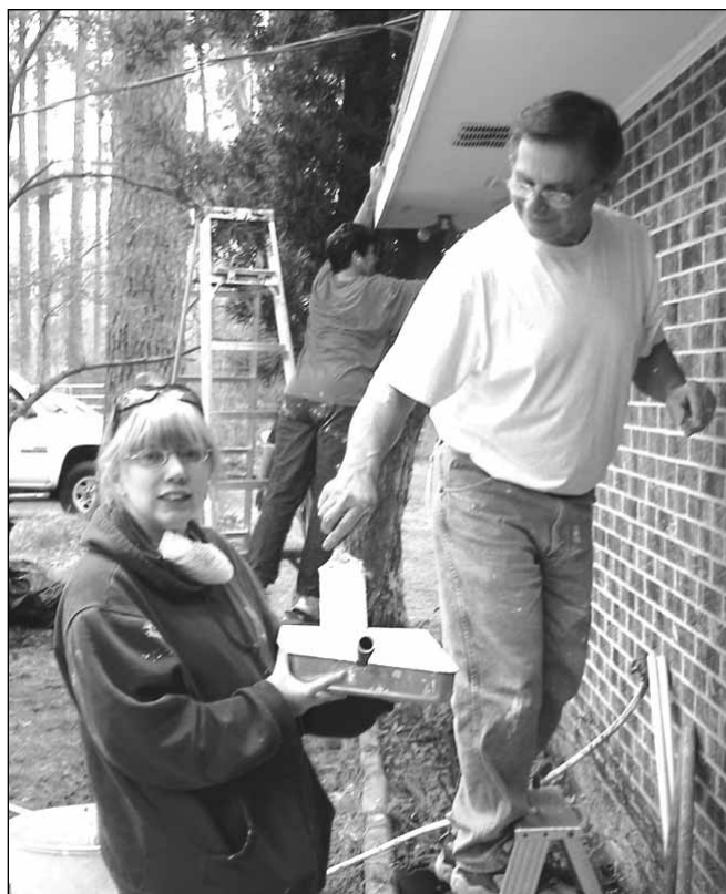
JESSICA HAHN, left, and Bob Bradford, right, work together to repair the hurricane-damaged home of Vicky Brooks during a recent mission trip to Louisiana. Terry Lighty is pictured in the background. All three volunteers are members of Saunemin United Methodist Church.
