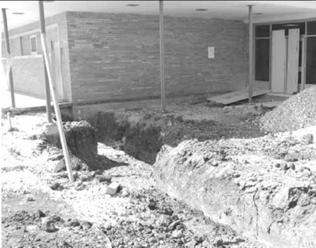
A NORMAL TRENCH that construction crews are digging for the footings of the DTHS cafeteria addition is quite a contrast from a nearby trench that is causing problems due to unstable ground. The problem trench is much deeper than this, as crews search for stable earth, and much wider, as its walls continue to collapse.
