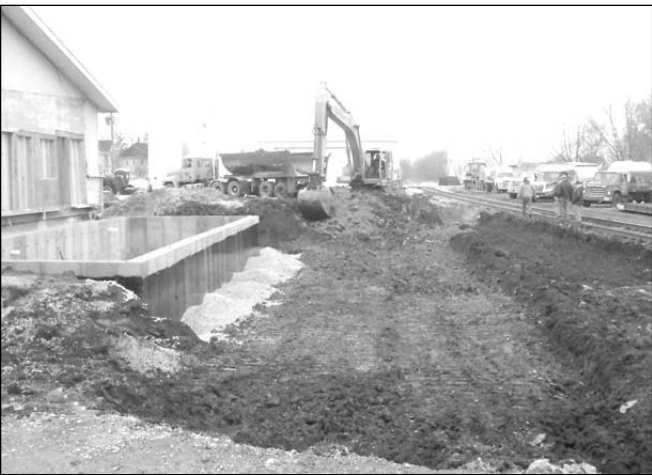
THE OFFICE/SCALE HOUSE at Herscher Grain was torn down, and a foundation for a new one was poured last week. The month-long project includes installing new scales, which can hold trucks up to 200,000 pounds – double the previous capacity. The new scales will be 75 feet long.
