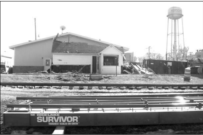
THE OFFICE AT HERSCHER GRAIN was torn down on March 3 to make room for the larger scales (in the foreground) to be installed soon. A year ago, the 130-year-old elevator was razed for the same purpose.
