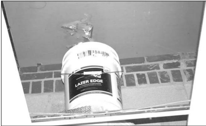
Above: A bucket sits below an area where water leaked in and damaged a ceiling tile in the freshman and sophomore hallway. A large screw missed the intended beam and instead went through the old flat roof causing the leak. Several classrooms and hallway areas throughout the second floor were water-damaged. Below: Workers put the finishing touches on a new green pitched roof that covers portions of the second floor of Dwight Township High School.
