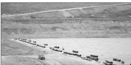
**LIVINGSTON LANDFILL** is building a new 13-acre cell on its site. On Friday, August 7, the facility led a bus tour past the new construction site, where a plastic liner is being laid to prevent water contamination by waste materials.
