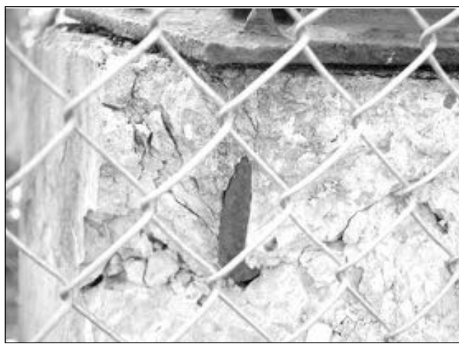
PILLAR OF SUPPORT — Dwight High School plans to replace the 45 concrete pillars, that support the football stands, which have begun to crumble and expose their rebar in the past several years.
