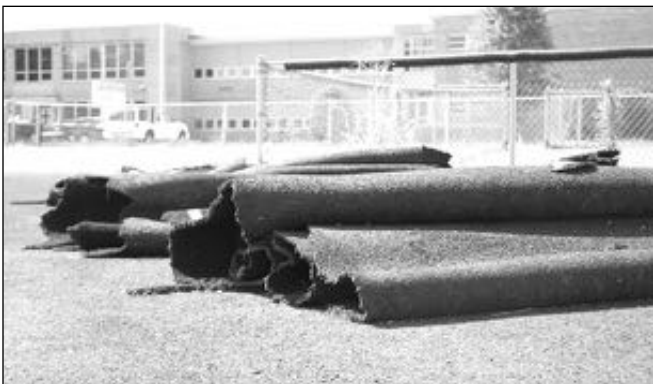
DWIGHT HIGH SCHOOL is giving its track a facelift as part of its summer maintenance. The school is laying new asphalt, after which one and a half inches of rubber (pictured above) will be overlaid.
