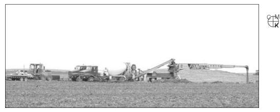
SEVERAL NARVICK BROTHERS TRUCKS dump concrete onto a conveyor that fills the large hole dug for the foundation of a wind turbine near 2600 East and 2200 North Road. They will deposit 55 truckloads of concrete into this hole for this one future wind
