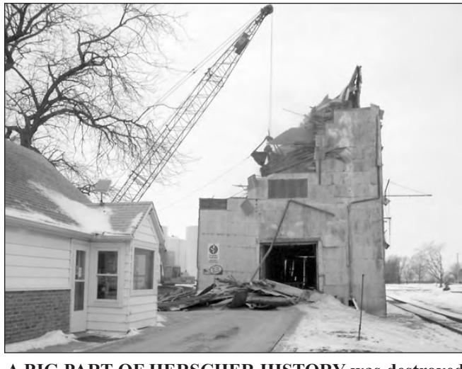
**A BIG PART OF HERSCHER HISTORY** was destroyed last week. The original part of the Herscher grain elevator, dating back to 1878, was torn down. It is believed to have been the oldest structure in Herscher, built four years before the village was incorporated. No replacement is planned for the spot. The elevator plans to extend its scales for trucks.
